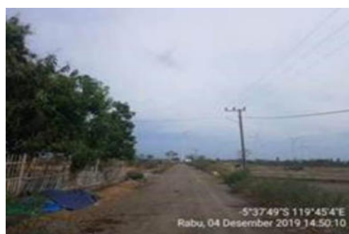
Road condition after repair
