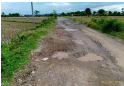
Road condition before repair
